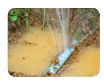
If the utility line is visible, keep the face of the shovel parallel with the utility line and use all precautions when removing the soil from around the utility line.
